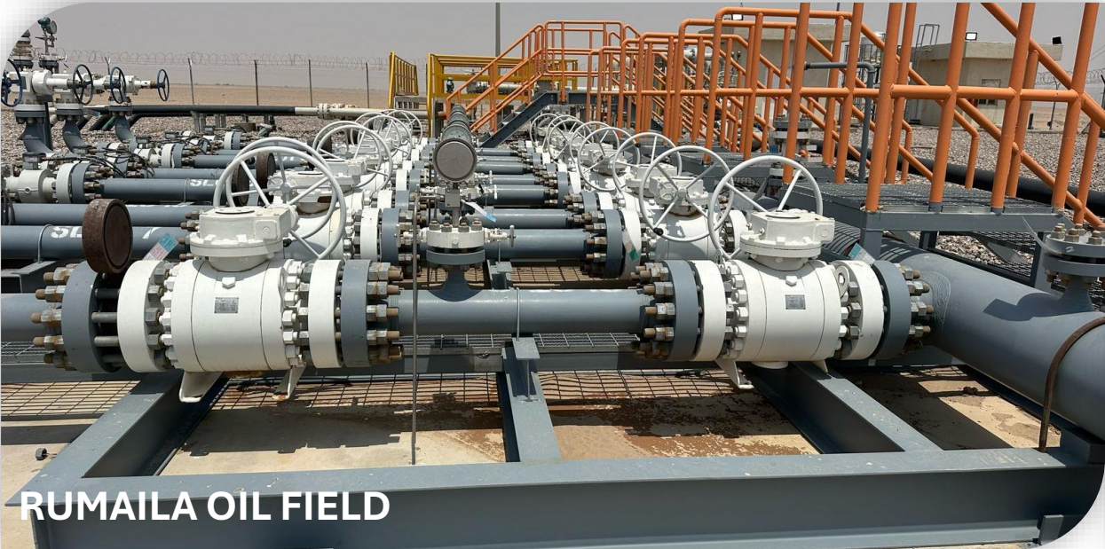
8 SLOT WATER INJECTION MANIFOLD
